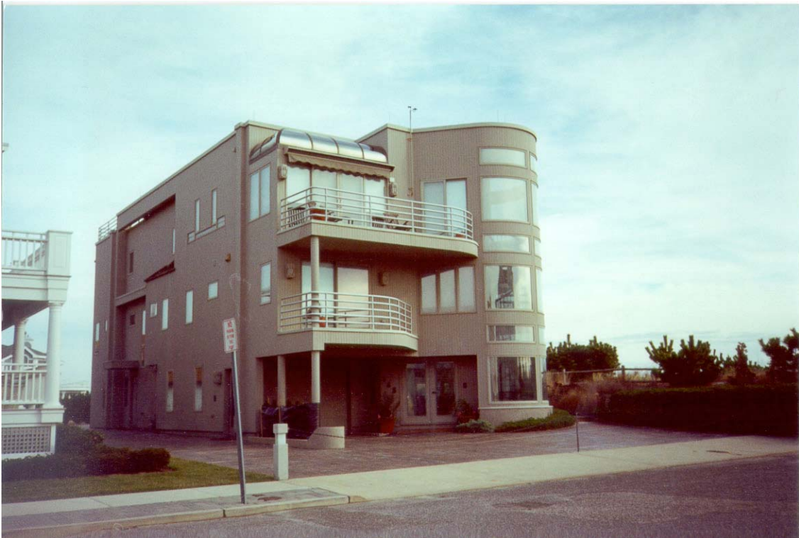
Three story dwelling with flat roof, surrounded by pavement, limited plantings, and one continuous curbcut.
