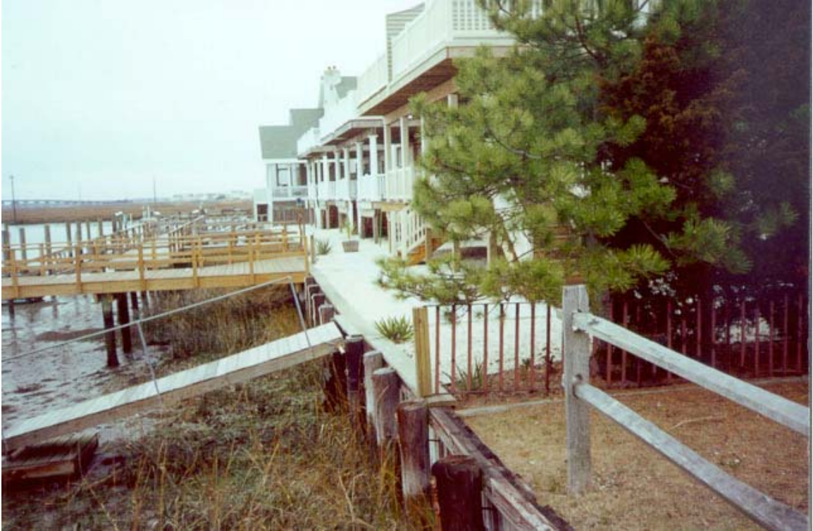
View west from the south end of 5 th Avenue. The second story decks in the foreground are approximately five (5) feet from the bulkhead line. Note the building in the background, which is constructed directly atop the bulkhead.
