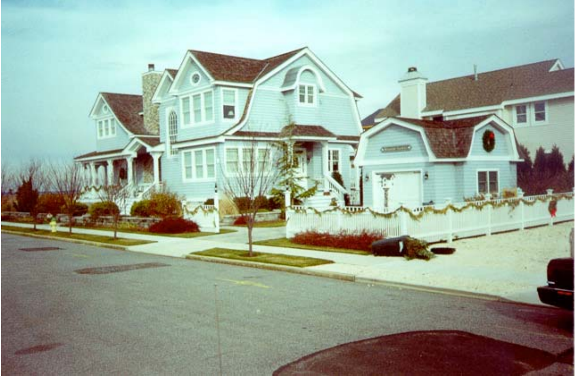
A new home constructed with architectural detailing including covered porches, chimney, decorative stairs, changing roof pitches, landscape plantings, and detached garage.
